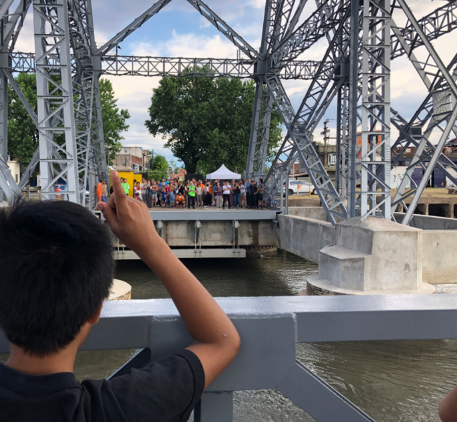
» FIG. 7.13 SPECIAL OPENING OF THE TRANSPORTER BRIDGE FOR THE NEIGHBORS OF ISLA MACIEL
